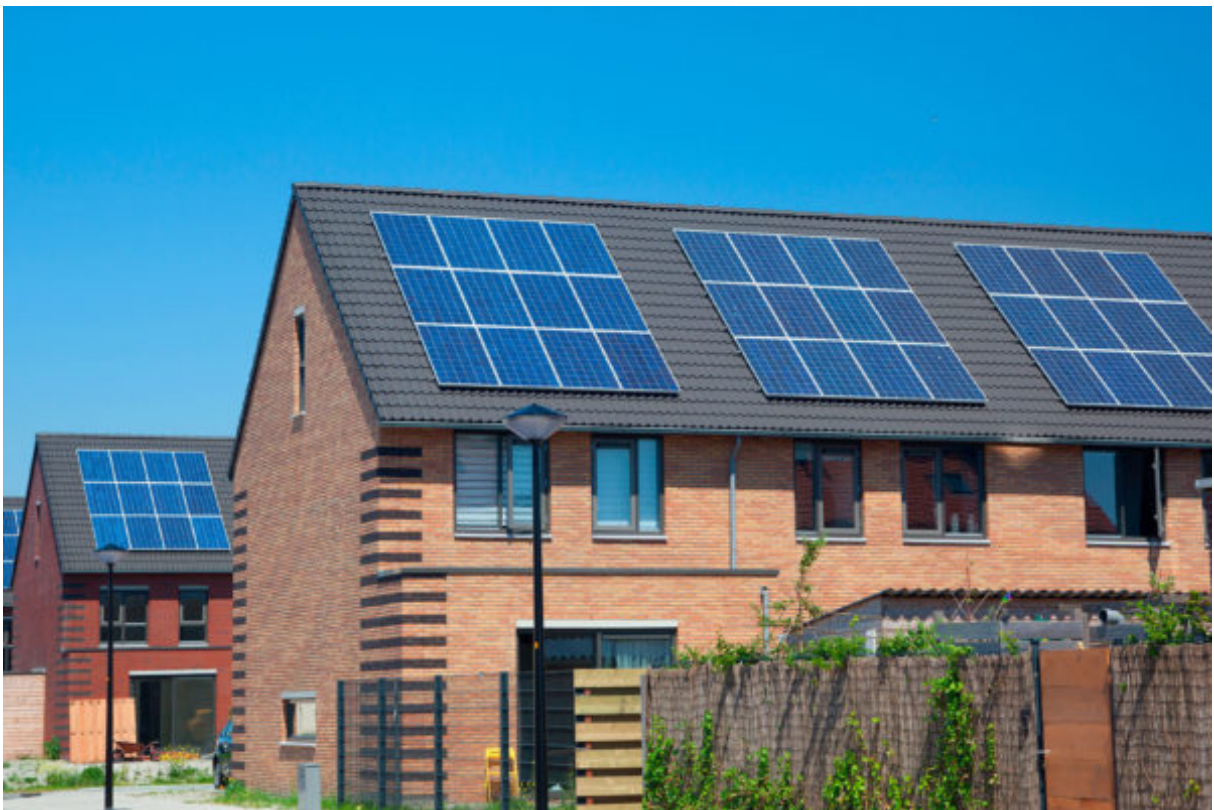
Picture 17: Solar panels installed in the roof of houses in UK (Gallucci, 2019)
