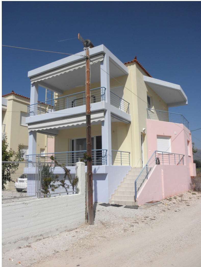
Picture 27: Building outside look
