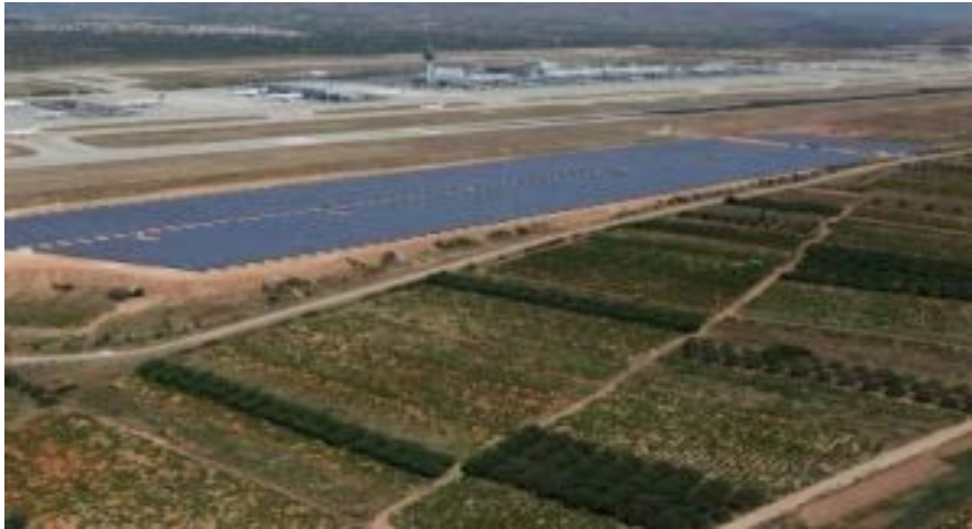
Figure 19. Aerial view of Athens International Airport PV farm installation (Greenair, 2012)
