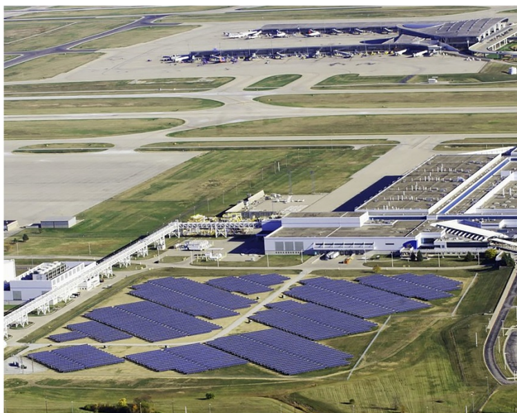
Figure 18. Fresno Airport PV farm installation (C&S Engineers, Inc., 2012)
