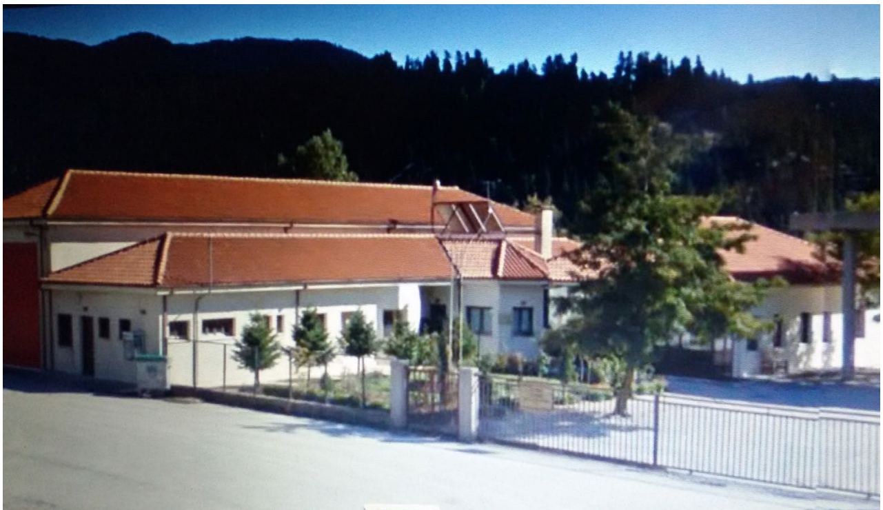
Figure 10: General View of the Investigated Building (Different Angle).
