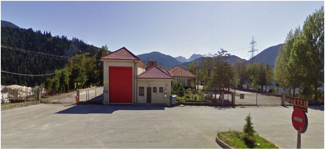
Figure 9: General View of the Investigated Building.
