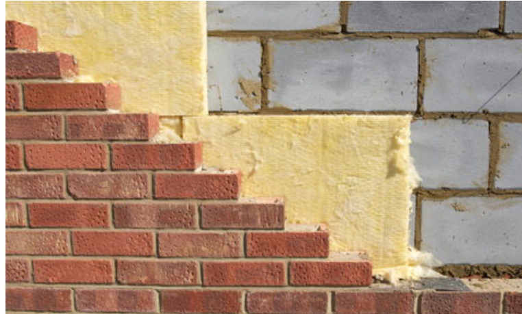
Image 17 Wall Insulation
