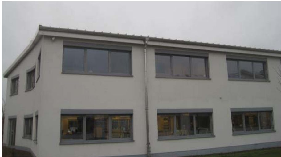
Figure 23: View of an office building from the side
