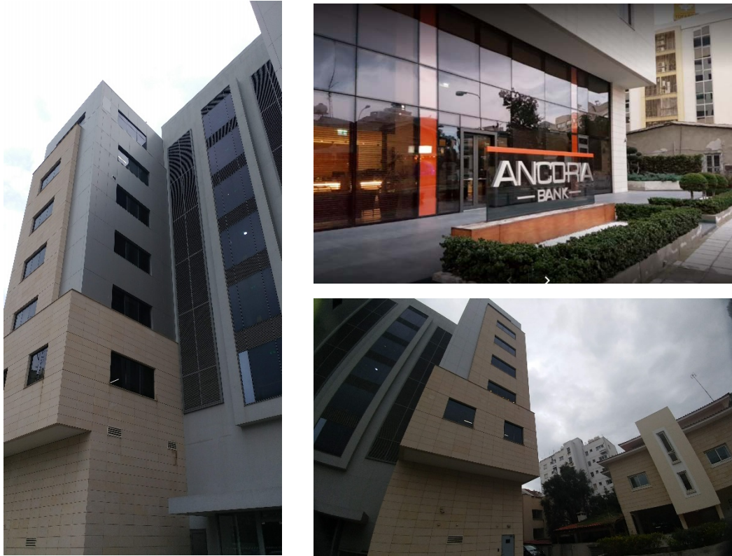
Photo 1 Different views of the building
