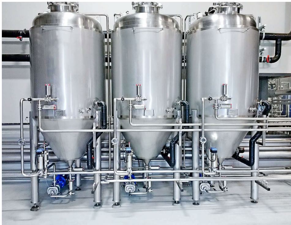
Picture 10 Yeast Propagation and storage tanks
