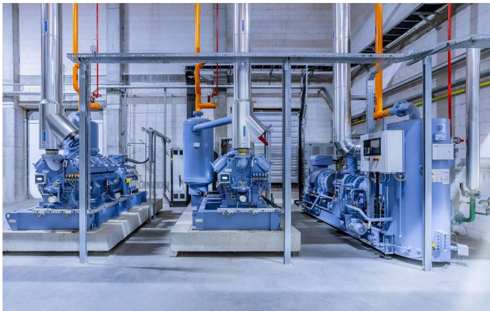
Picture 17 NH3 Compressors (GEA refrigeration solutions, 2020)
