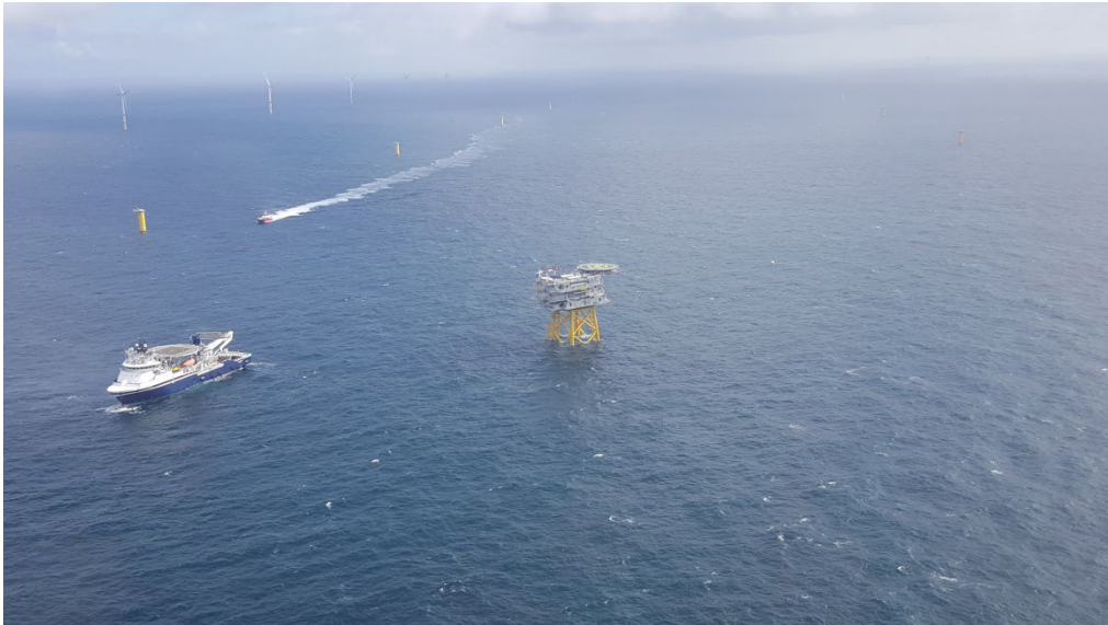
Figure 7 Sandbank OWF under construction
