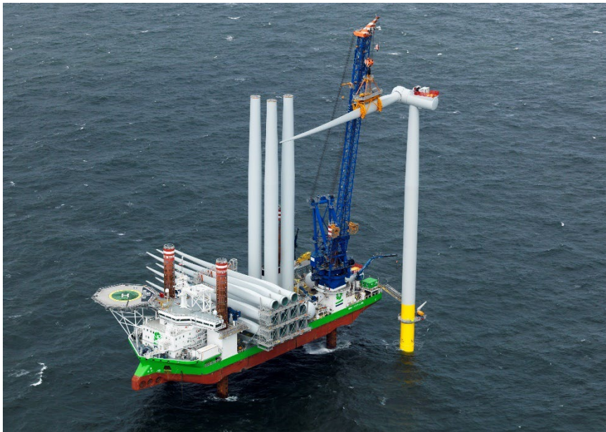
Figure 11 Installation of a wind turbine in Borssele 1+2
