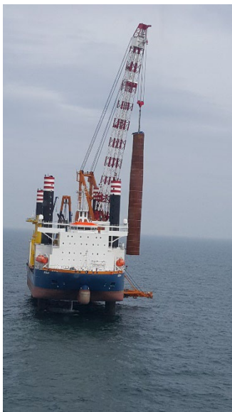
Figure 4 Installation of a monopile in Gemini Offshore Wind Farm
