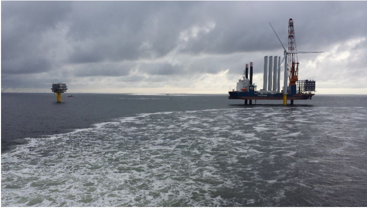
Figure 5 Installation of a wind turbine in Luchterduinen Offshore Wind Farm
