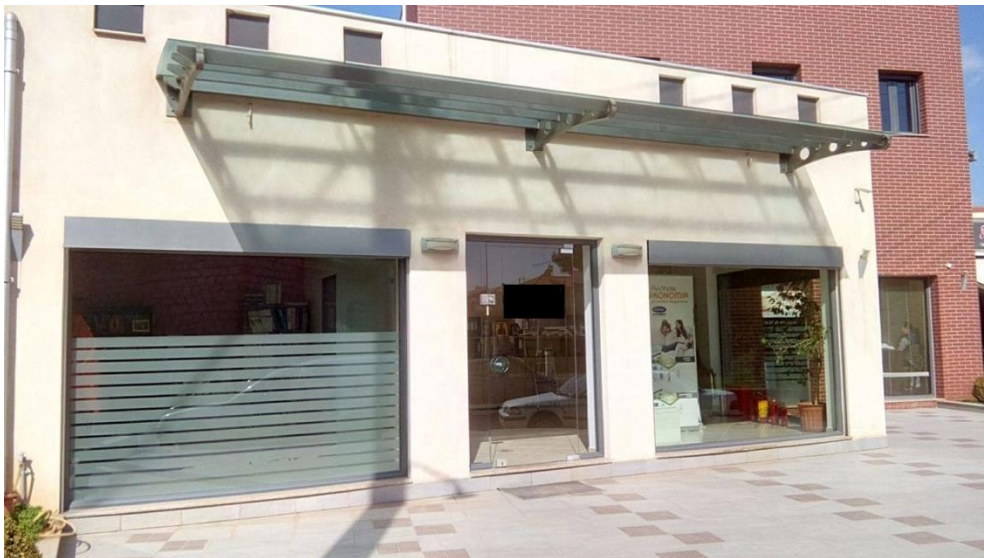
Figure 7: Façade of the examined office
