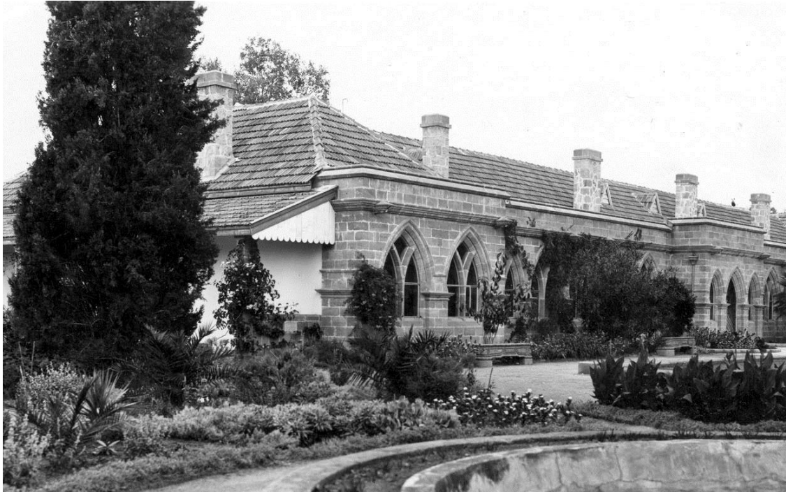
View of the Government House before the October events, 1931 (Image courtesy of the Press and Information Office, Republic of Cyprus).
